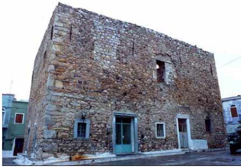
Figure 2. Photograph of an old building.
